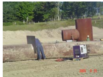
Welding anti-seep collars to pipe
