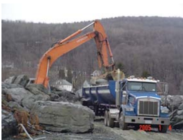
Silverline Construction loading rock onto to Mix Brothers truck
