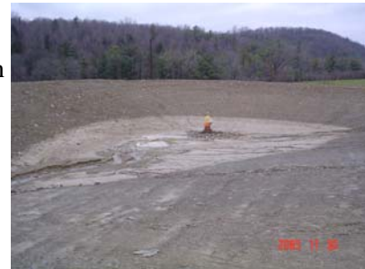
Finished pond with riser
