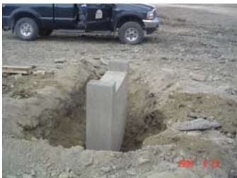
Pipe bent complete
