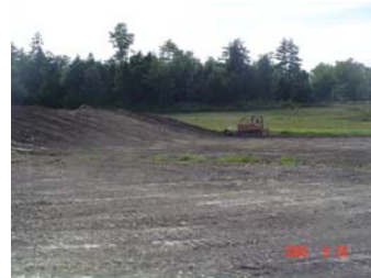
Stripping topsoil
