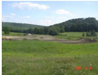
Starting to strip topsoil
