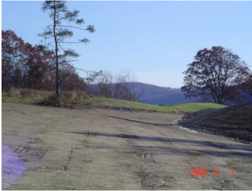
Diversion ditch under construction
