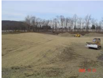
Gravel pit sides were sloped and seeded
