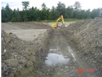
Digging the core trench
