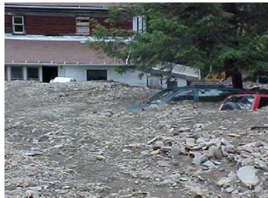
The babbling stream became a residential nightmare. Gravel is up to the middle of the 1st floor and the cars are nearly buried
