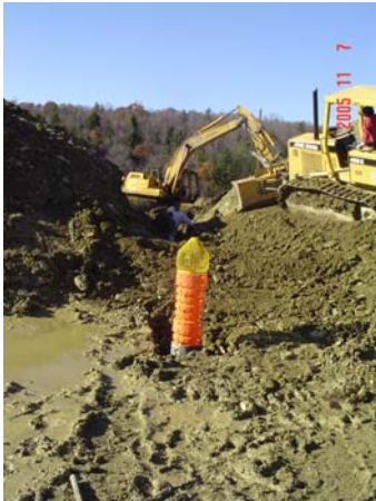
Installing pipe & anti-seep collars for outlet
