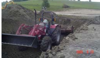
Compacting the core trench
