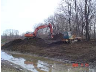
Silverline Construction & Hendershott Excavating working on channel
