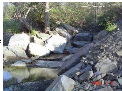
Rock used to pave the outlet of this road culvert
